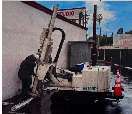
Small Rig - Direct Push Technology Used in Initial Attempt
