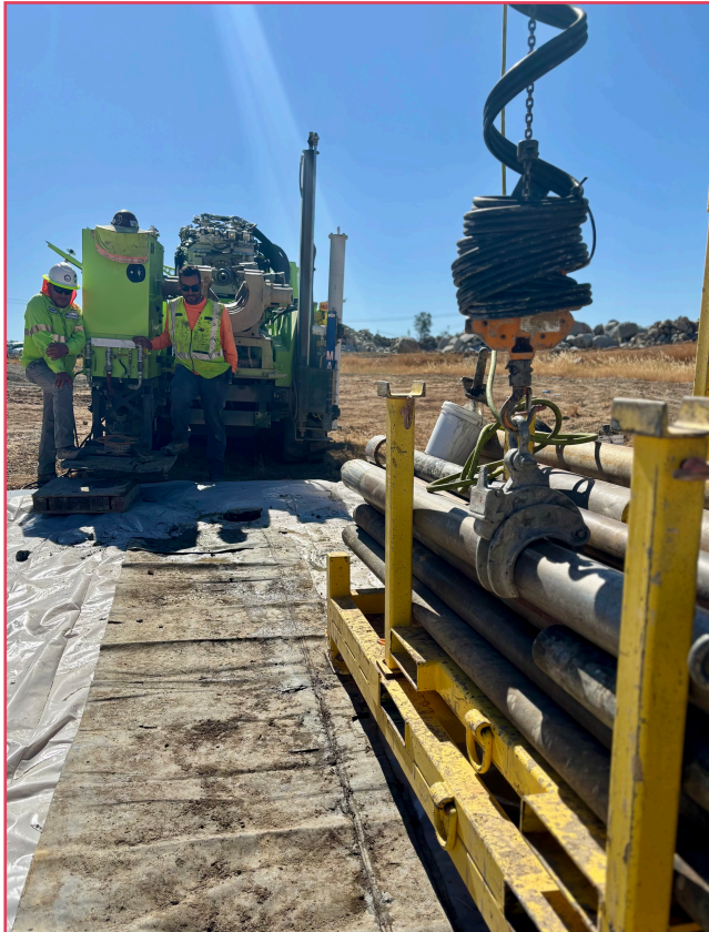
Workers in August tested one possible remedy using a large sonic drill to inject a compound to try to neutralize the TCE. (Photo by Maj. Kara Greene, USACE)
