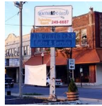
Abandoned or dilapidated signs
