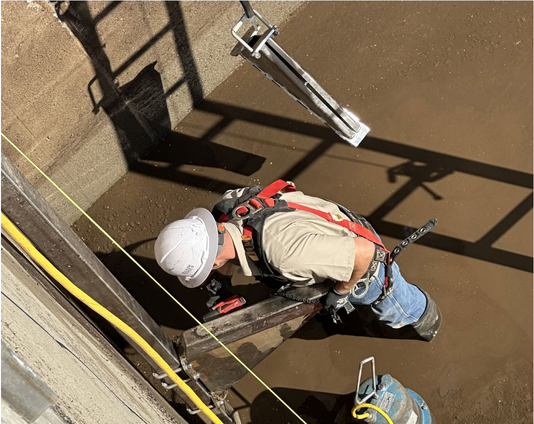
Photo 2: Ditch#2 Anoxic Mixer 2B Repair
