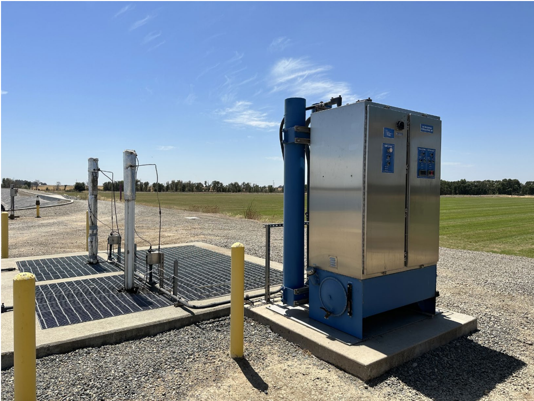
Photo 4&5: Before and After Beck Actuator Installation
