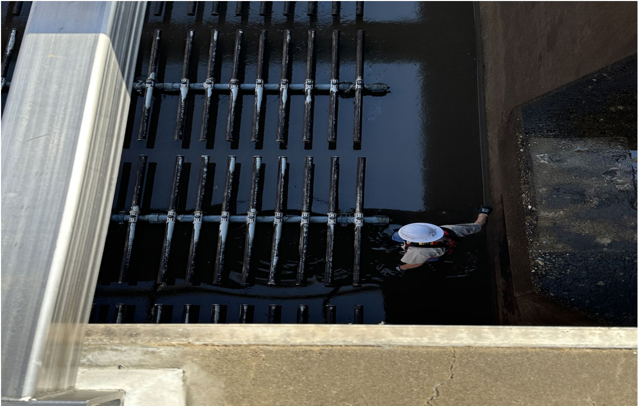
Photo 3&4: Ditch #2 Diffuser Replacement Before and After
