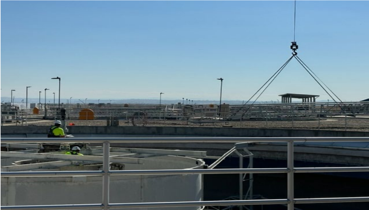
Photo 4: Clarifier Drive replacement. Note cat walk suspended from crane.
