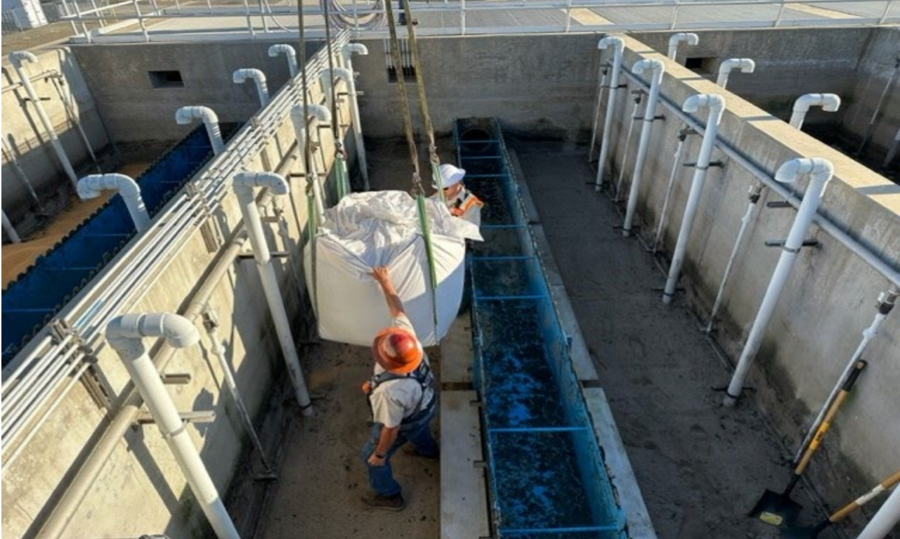
Photo 2: Filter sand addition
