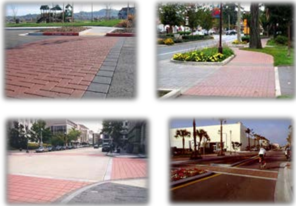
Enhanced Intersection with Decorative Paving
