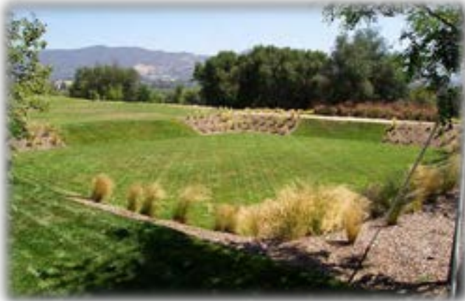
Image of Built Detention Basin
