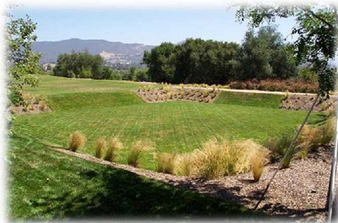
Image of Built Detention Basin
