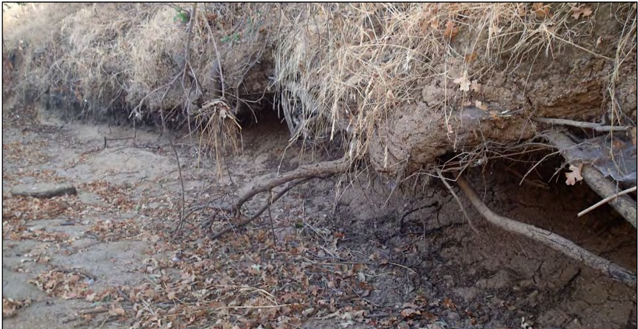
Photograph 8. Representative bed and bank of Markham Ravine, depicting scour as indicator of OHWM.
