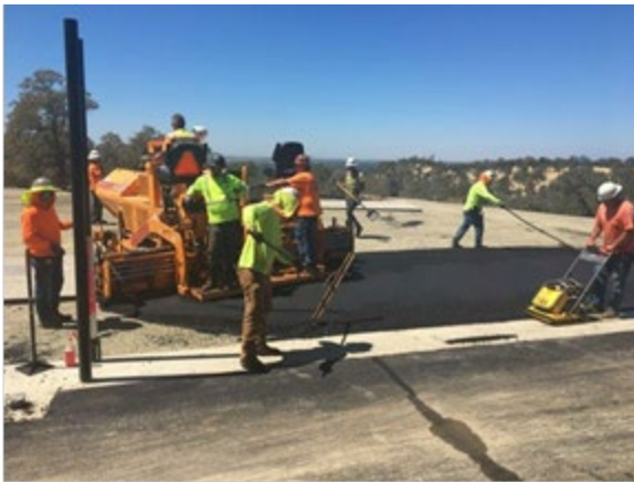
Paving at westerly gate to metering station.
