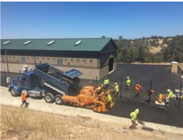
Paving along easterly side of metering station.
