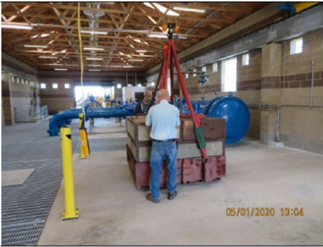
Load testing the overhead traveling crane inside the metering station.
