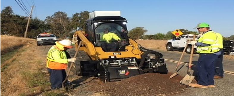
Streets Crew at work repairing Moore Rd with the new skid-steer planer. The new planer is fast, efficient and surprisingly quiet to use. It makes removal of damaged pavement much easier and more accurate than using a jackhammer.
