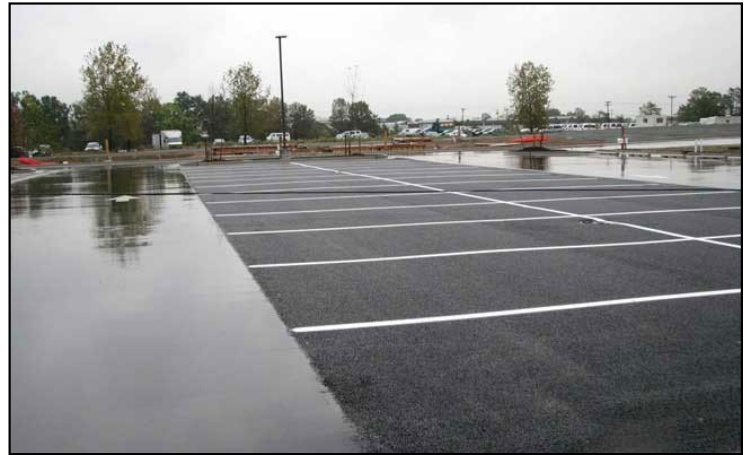
Permeable pavement. Source: EPA
