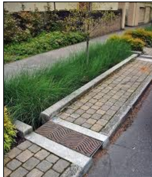
Roadside bioretention. Source: sitephocus.com
