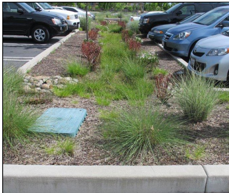
LID vegetated swale parking lot. Shellito Indoor Pool, Roseville. Photo: Greg Bates
