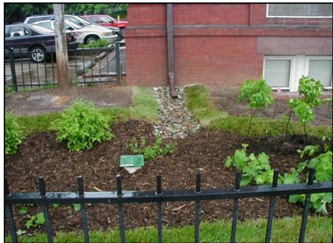
Rooftop disconnection. Source: LID Center
