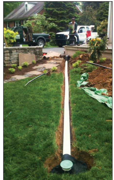
Bubble-up emitter installation. Photo Source: green-weaver.com
