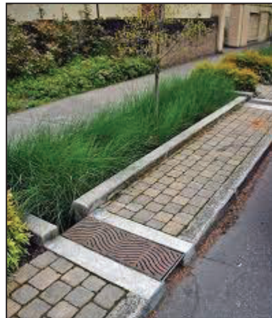
Roadside bioretention. Source: sitephocus.com
