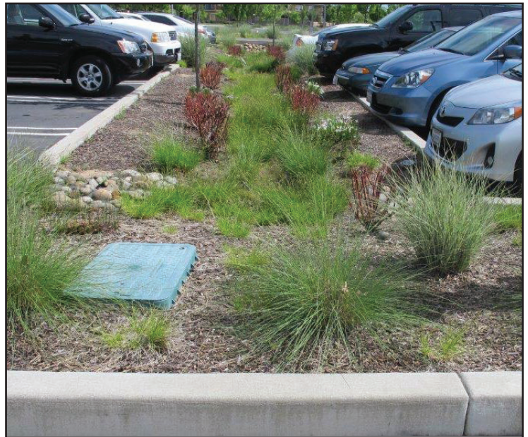
LID vegetated swale parking lot. Shellito Indoor Pool, Roseville. Photo: Greg Bates
