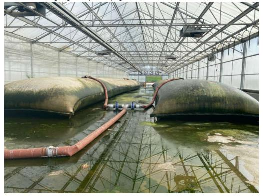
3. Bags removed and biosolids drying with "moles" turning over material.
