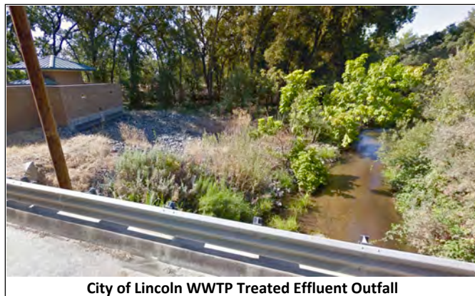
City of Lincoln WWTP Treated Effluent Outfall
