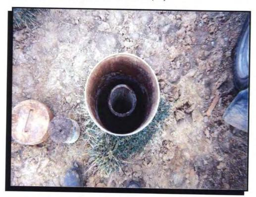
Photo 20: Close-up of City of Lincoln four-inch monitoring well casing.
