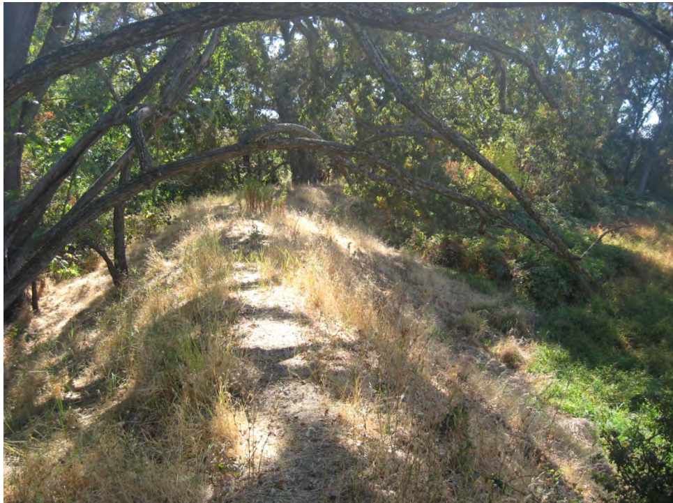
View of Auburn Ravine levee looking south
