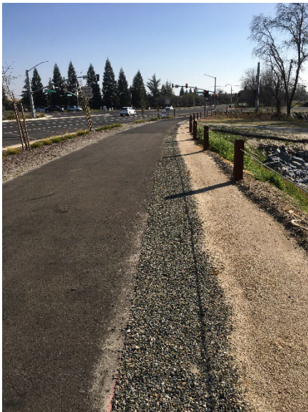
Photo 7. Ferrari Ranch Trail east of Auburn Ravine Natural Preserve Area, facing south toward McBean Park Drive/Ferrari Ranch Road intersection
