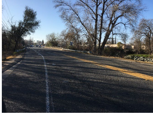
Photo 6. McBean Park Drive at Auburn Ravine, facing west
