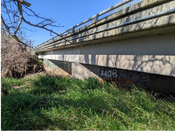
Photo 5. McBean Park Drive over Auburn Ravine Bridge, facing northwest
