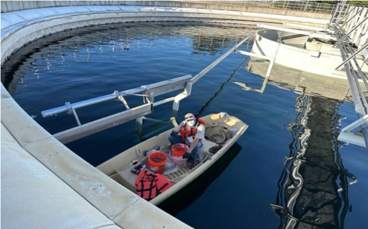
Photo 3: Clarifier #2 Skimmer Arm Coating
