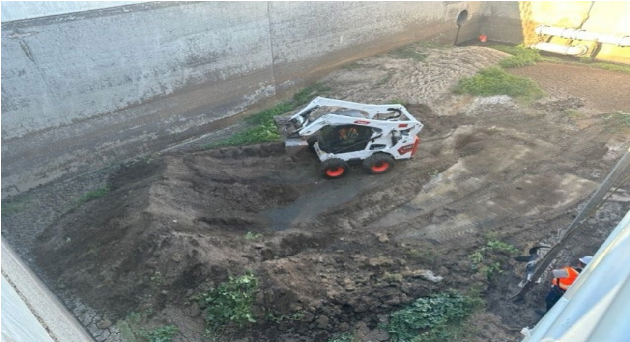
Photo 2: Ditch #3 Grit removal
