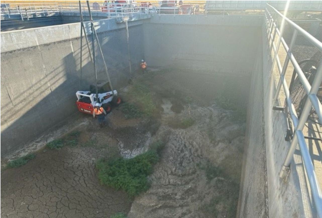
Photo 2: Ditch #3 Grit removal
