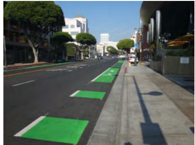
Figure 27: Example Green Colored Pavement Markings
